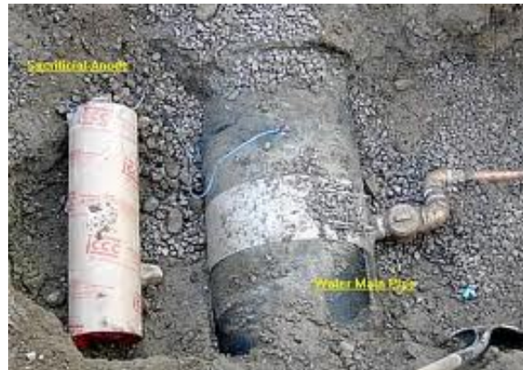
Image of Sacrificial Anodic Protection
